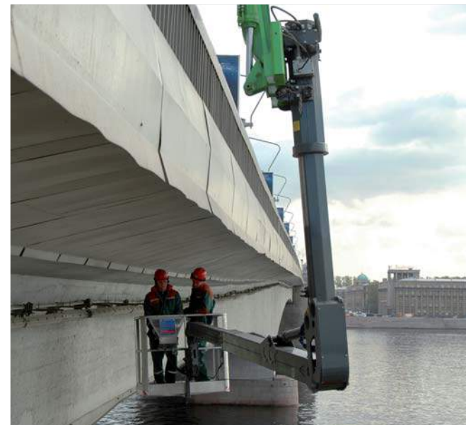
The Space System makes it possible to operate at a negative level of over 9 meters below street level
